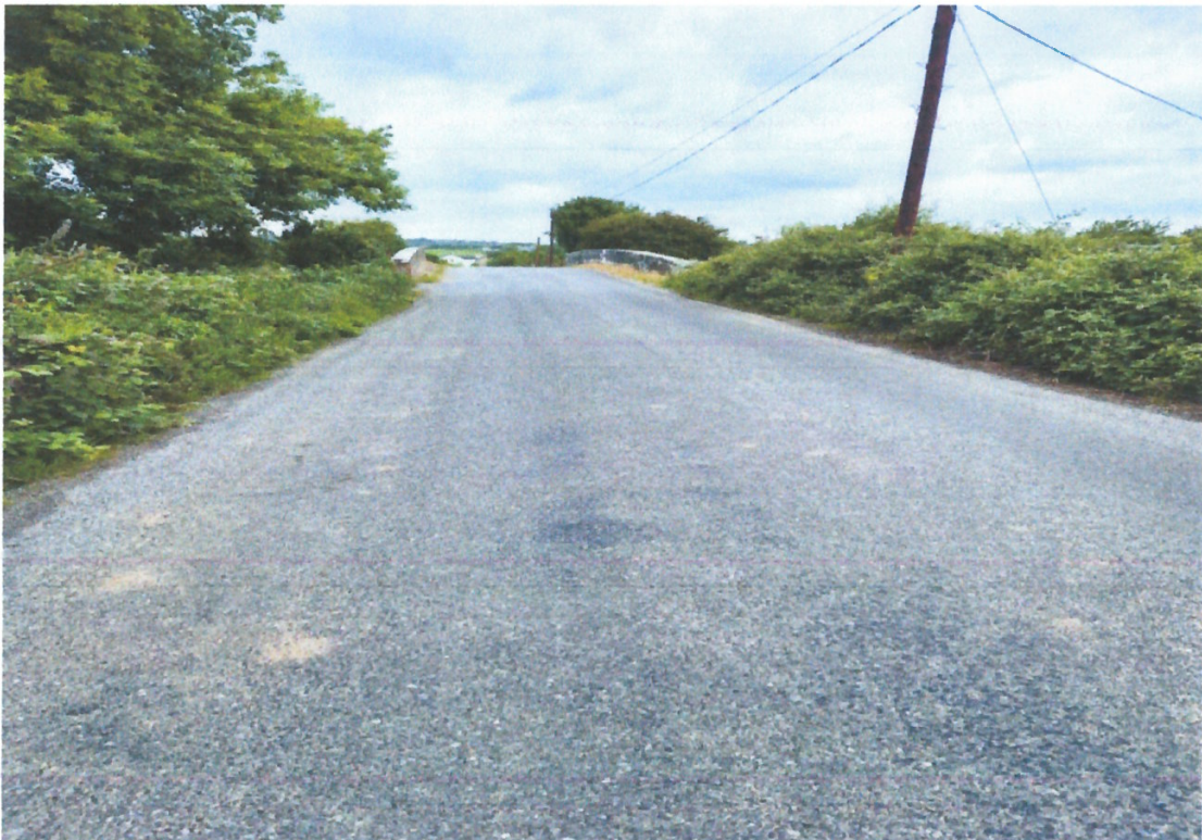
Fig 7.4 Grange Bridge looking West
