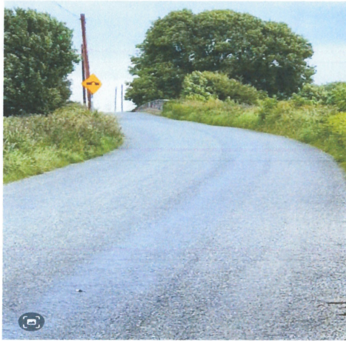
Fig 7.3 Grange Bridge looking East.
